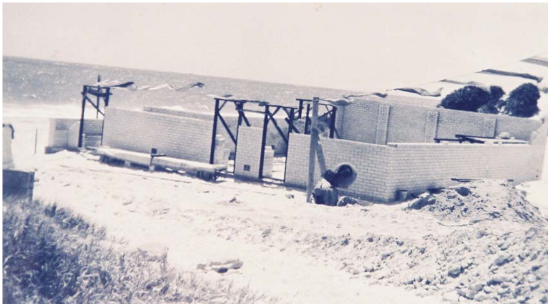
Construction of Sorrento SLSC 1960
